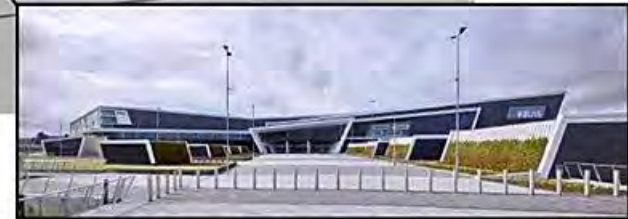
Landscaped Podium Deck with Undercroft Car Park
