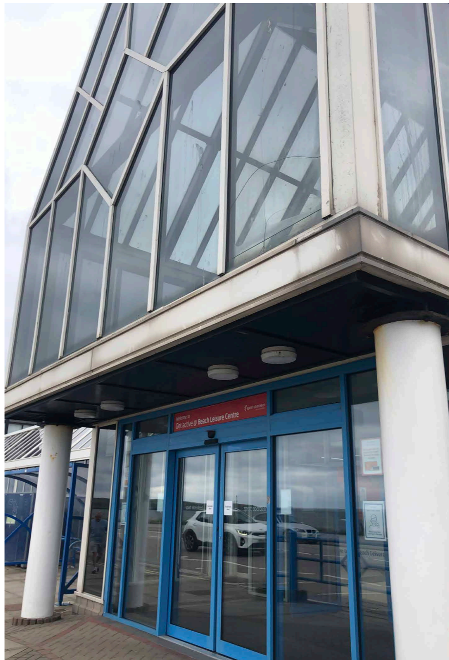
Existing entrance to Leisure Facility
