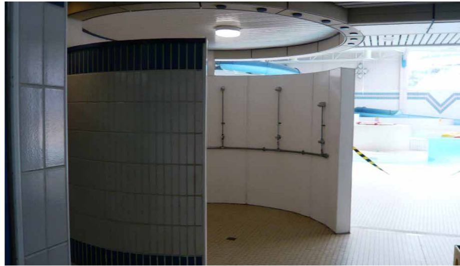
Existing shower in swimming facility
