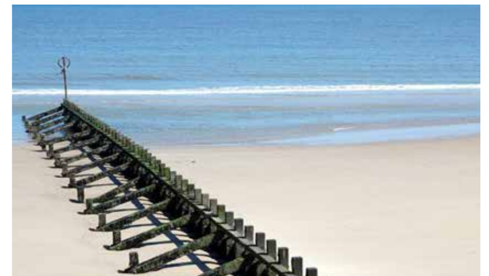
Image of the groynes structures which are positioned along Aberdeen Beach
