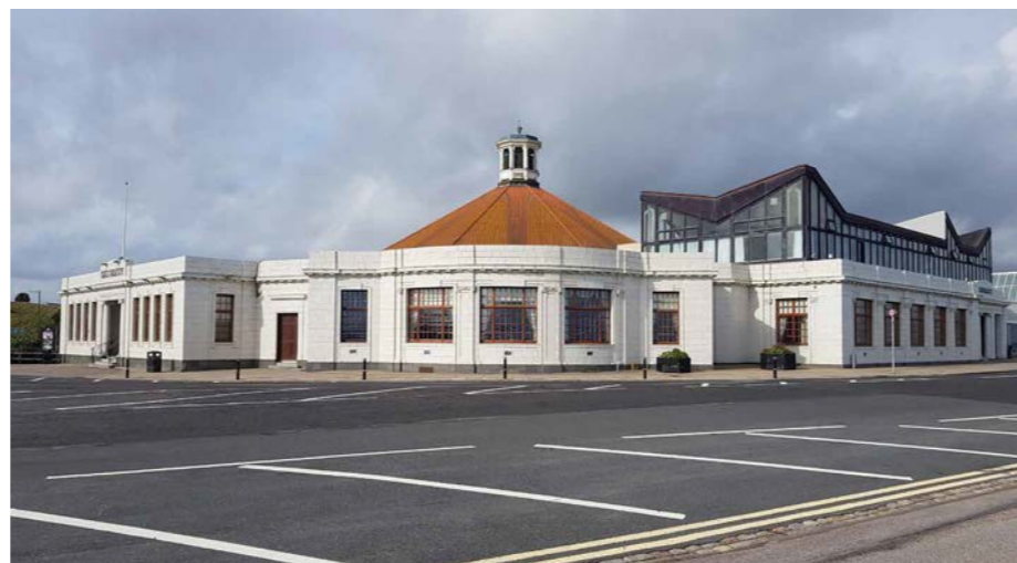
View looking towards Beach Ballroom
