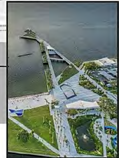
Dynamic pier structure extending out from existing linear Groyne with focal viewing platform
