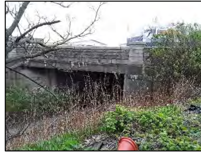
Photograph 14: Bridge structure with gaps providing PRFs in the site
