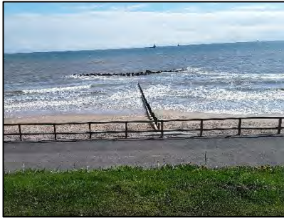
Photograph 11: Groyne and wooden posts along beach for support and protection
